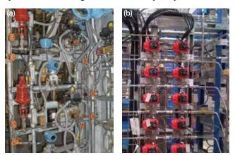
▲ Figure 4. (a) Banks of valves and instrumentation installed with metal tubing and electrical conduit are expensive and difficult to alter if additional equipment or connections are needed. (b) Valves connected via plastic air lines and push-type quick-release fittings are less expensive, easier to install and change, and do not compromise safety.
